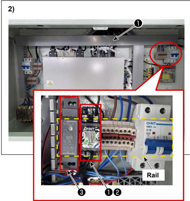
2) Attach RELAY ① , RELAY TERMINAL ② and BK10\_24V\_POWER\_SUPPLY ③ to the rail located at the upper right section of the electrical rack.
