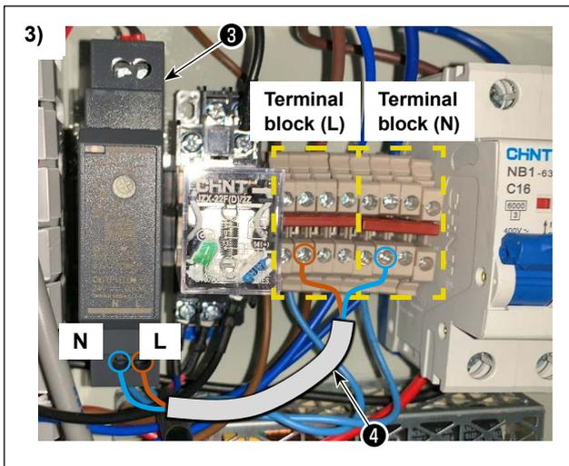
3) Connect BK10\_24V\_POWER\_SUPPLY ③ , terminal blocks (L) and (N) with BK10\_24V\_POWER\_CABLE ④ .
