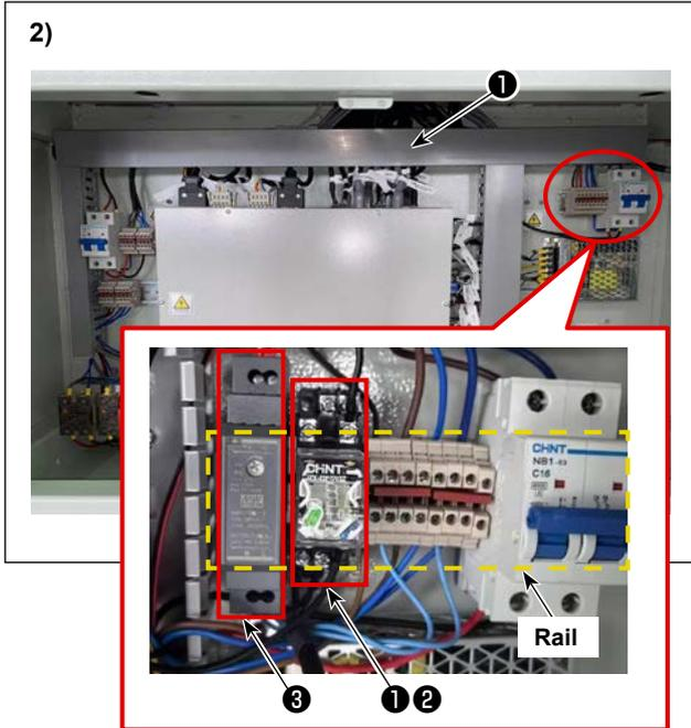
2) Attach RELAY ❶ , RELAY TERMINAL ❷ and BK10\_24V\_POWER\_SUPPLY ❸ to the rail located at the upper right section of the electrical rack.
