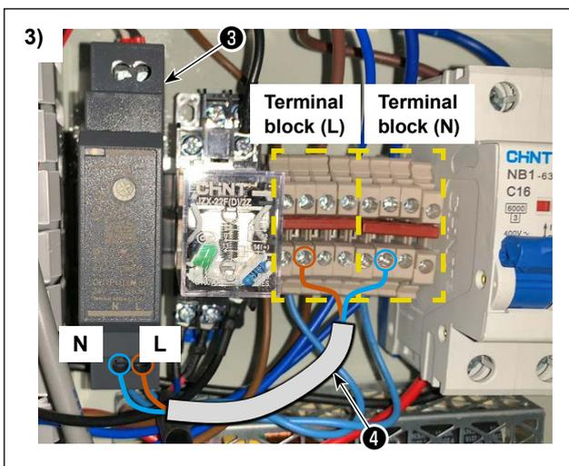
3) Connect BK10\_24V\_POWER\_SUPPLY ❸ , terminal blocks (L) and (N) with BK10\_24V\_POWER\_CABLE ❹ .
