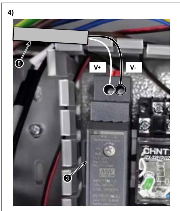
4) Connect power cable ⑤ of the BK control box that you have drawn into the electrical rack in Steps ④ to ⑦ to BK10\_24V\_POWER\_SUPPLY ③ .
