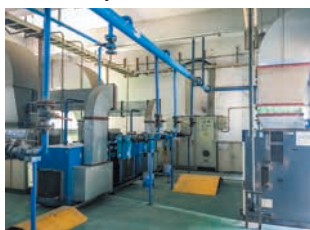
Five fixed-frequency compressors (295kW total)
