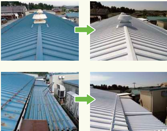
Some roofs of the factory aged by corrosion were changed to those that had been painted with heat insulators.
