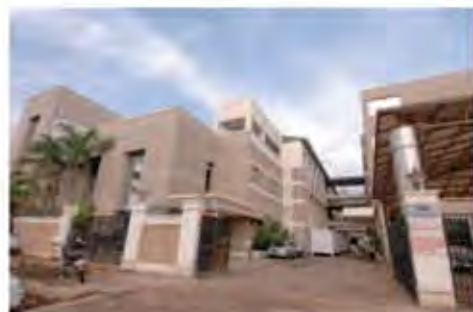
Front view of the plant
