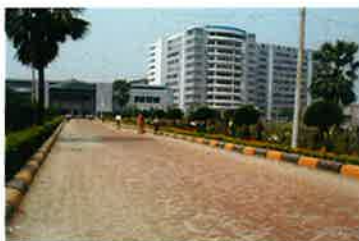
Front view of the plant
