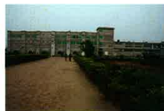
Front view of the plant.
