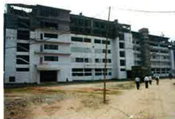
The new plant under construction. Expansion is made at full speed to meet the yearly growth of the business.
